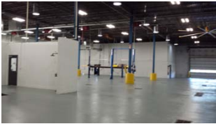
Coatings Single Broadcast @ City Mechanic Shop
