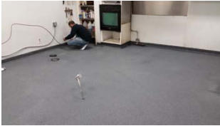
Coatings Double Broadcast Kitchen Floor
